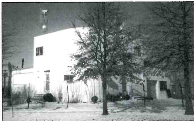
The WEEI transmitter building as it looks now. (Courtesy Richard Amirault, N1JDU.)
